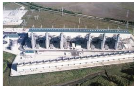
Forney Power Plant Source: NextEra Energy
